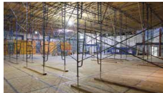
Indoor shot of the seismic work at Newport High School gym.
