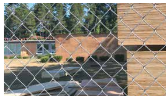
Outdoor shot of the seismic work at Sam Case Elementary.
