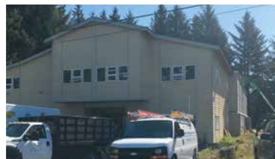
Renovation of the old pool into the Teaching and Learning Center.
